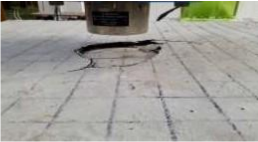
Fig. 15. Crack Pattern on Bottom of Slab
