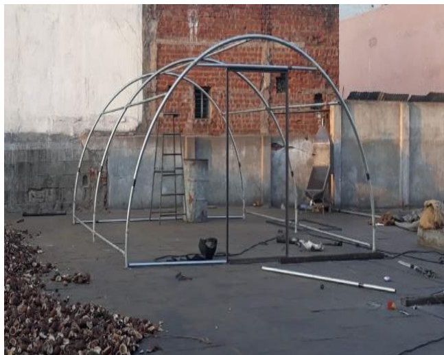
Fig.1. Frame work of solar Tunnel dryer
